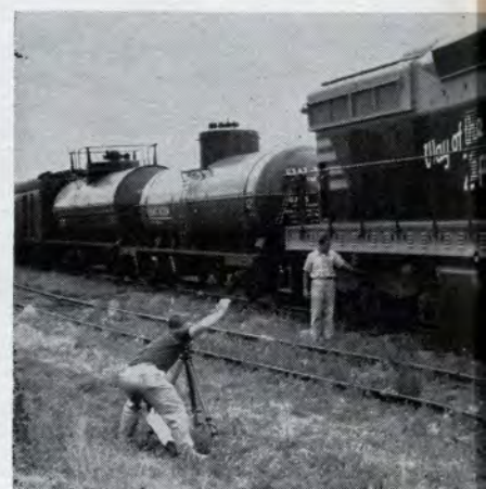
A team of engineers from Boeing check the settling rate at this particular siding. How much the track sinks under a heavy load could affect the aiming formula for the ICBM at this site.
