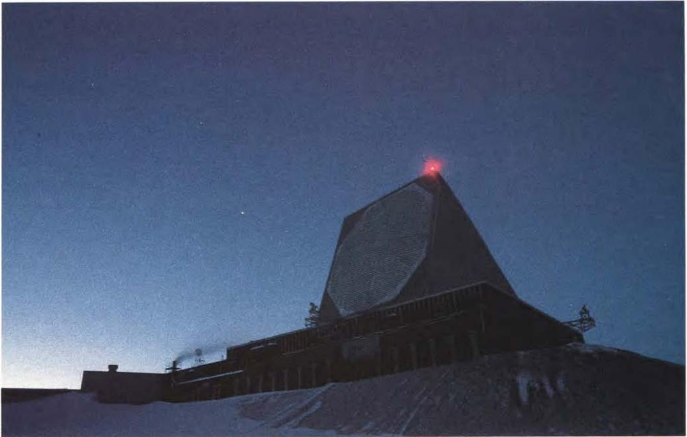
dar to Thule in 1961. The upgraded version, which Raytheon installed at a cost of \$110 million and now helps maintain, is a two-sided, electronically steered, phased-array sensor that can do a vastly better job of detecting, tracking, and assessing ICBM launches than could the three mammoth radar dishes that made up the old system.
