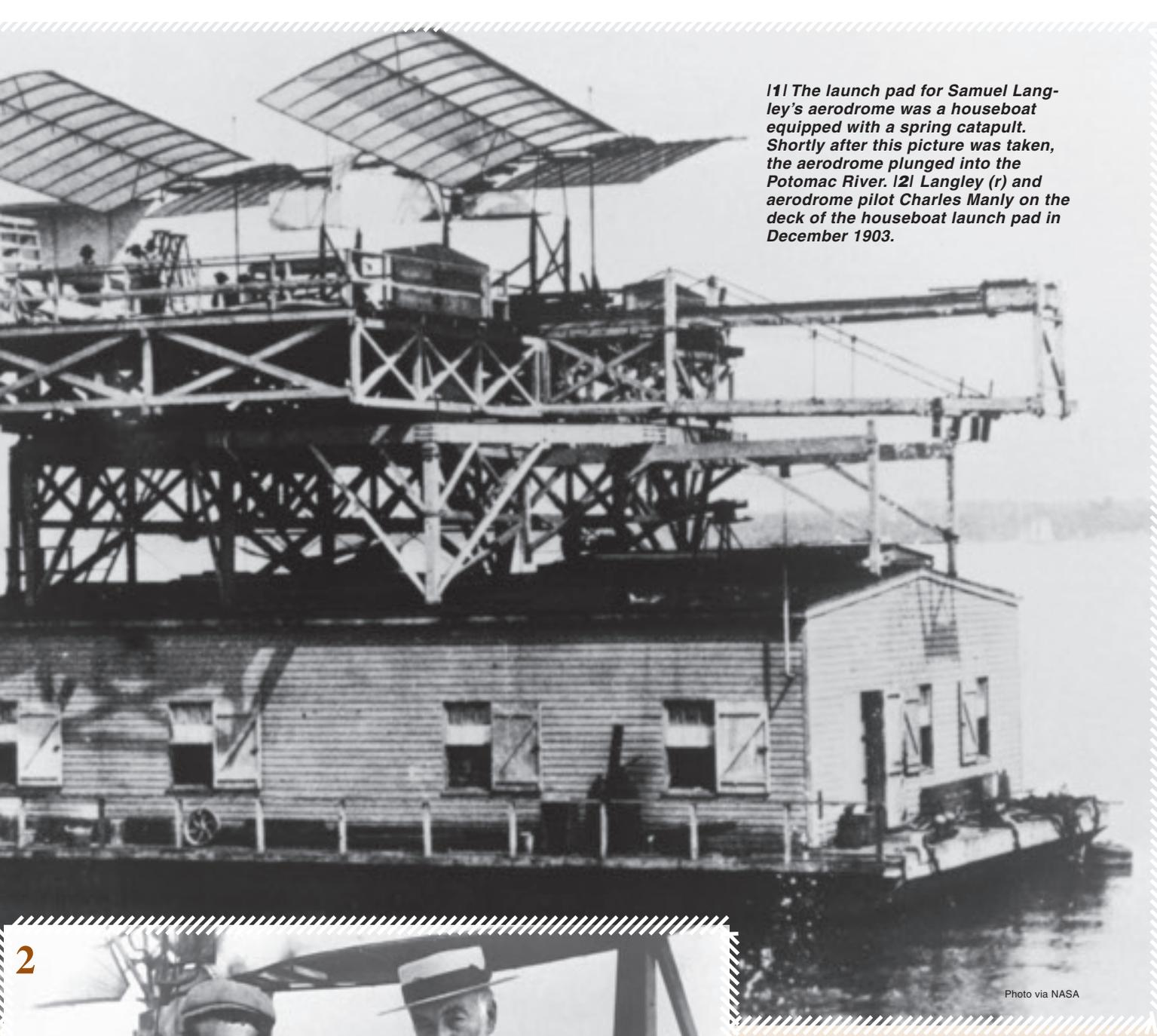
**111** The launch pad for Samuel Langley's aerodrome was a houseboat equipped with a spring catapult. Shortly after this picture was taken, the aerodrome plunged into the Potomac River. **121** Langley (r) and aerodrome pilot Charles Manly on the deck of the houseboat launch pad in December 1903.
