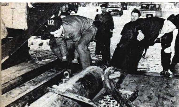
Alaskan Air Command and Civil Defense personnel pitched in to keep supplies moving during the post-quake period. Above, a crew of military people and civilian volunteers work together in biting cold at Seward to unload aid cargo from a C-123 Provider. Supplies were rushed to needy areas.
