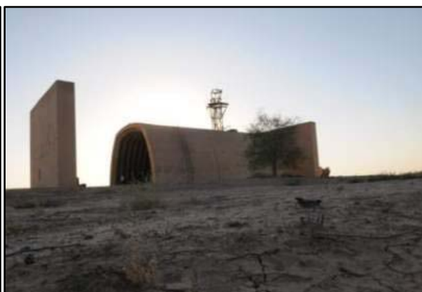
Figure 10: Side View of Structure
